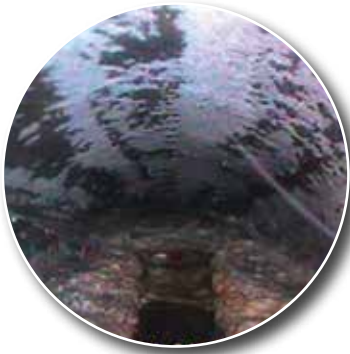
View of FOG build-up inside sewer pipe
